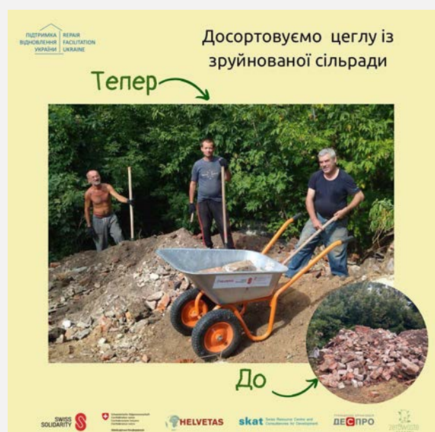
Efforts at the Circular Construction Yard in the Kharkiv region.
